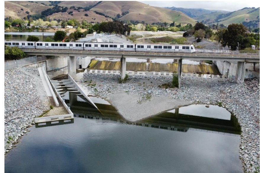
One of ACWD's fish ladders as part of the Fish Passage Improvements Program.
