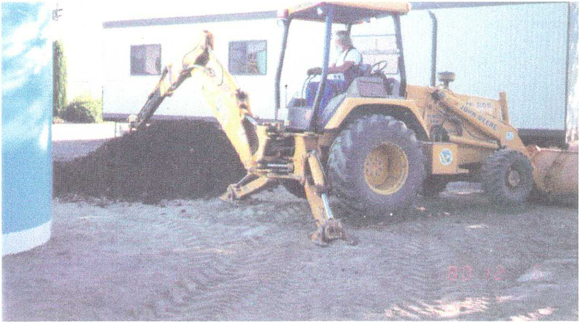
The peat soil was mixed by a backhoe prior to loading into the tanks.
